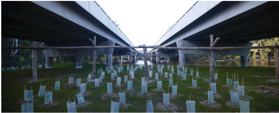
Pacific Highway, Bonville Upgrade Project Image Courtesy of Abigroup Limited
